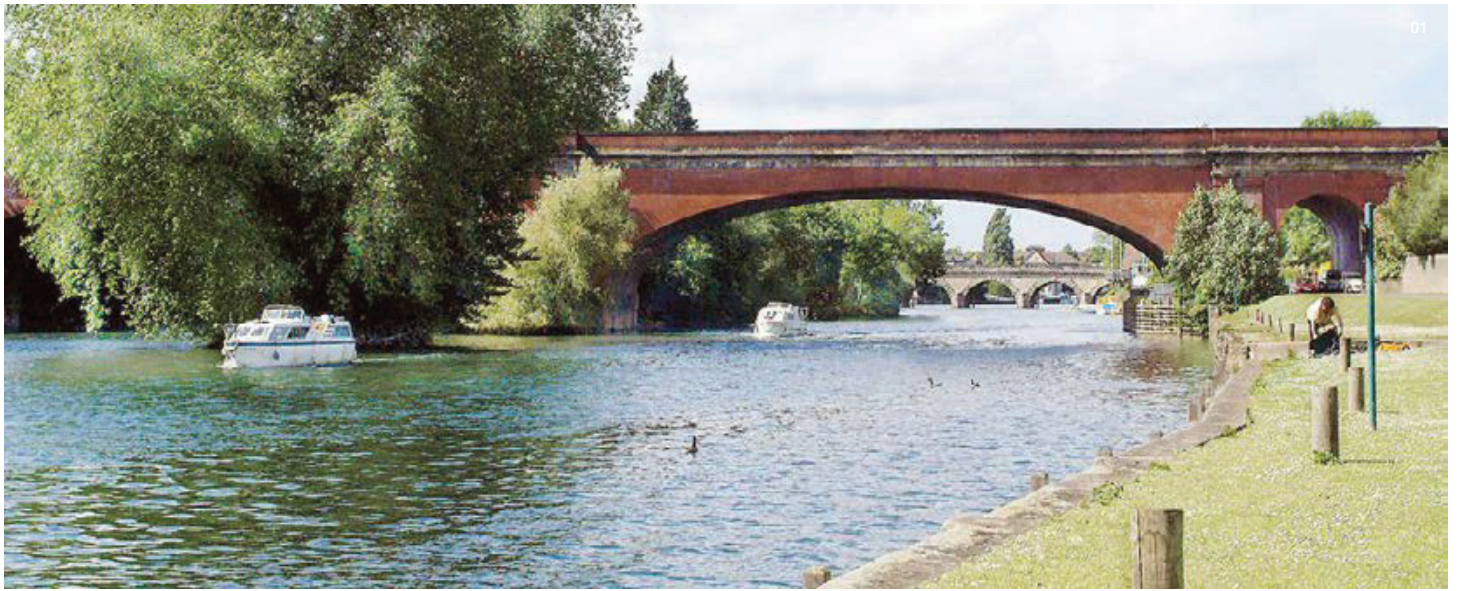
01 Brunel's Sounding Arch, Maidenhead 02 Stanley Spencer Gallery
